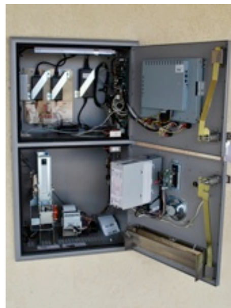
Stainless Steel construction to match the elements.
